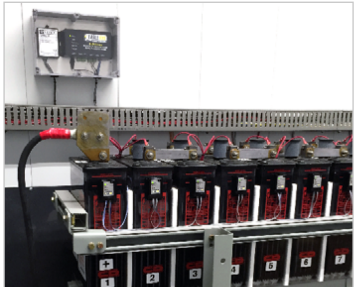
Installation to Battery Cells
